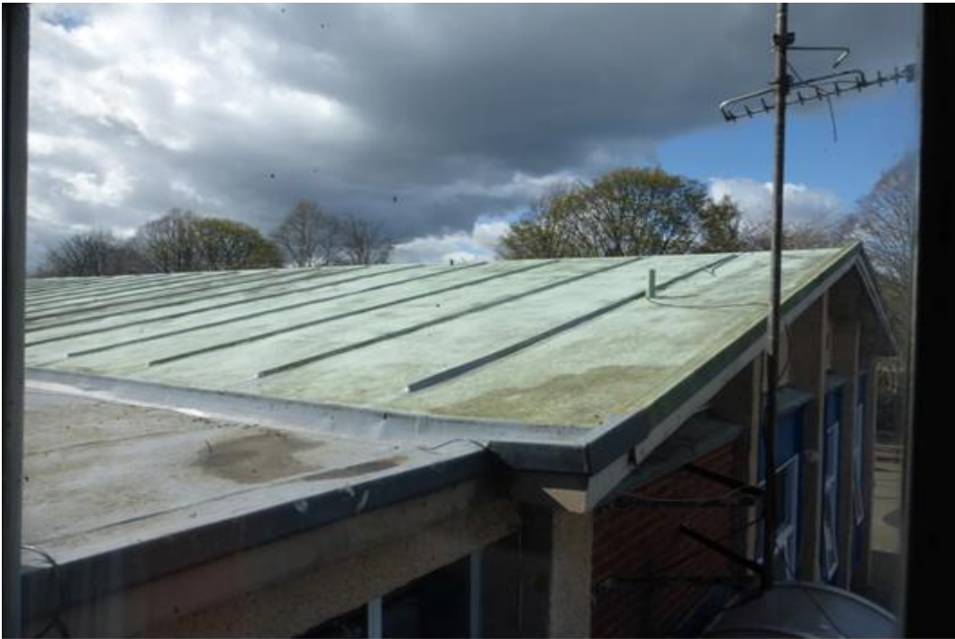
Photograph of Clermiston PS roof before enhancements
